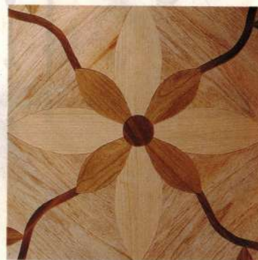
Details of the computer-cut sections of the floor with strip accents and the finished flower motif.
